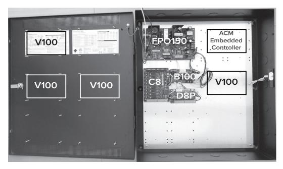
Install the ACM Embedded Controller and V100 subpanels as shown below:
